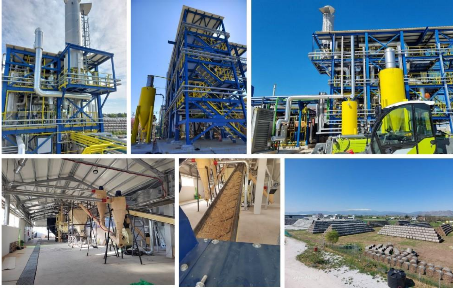
AGRIGAS 500 kW gasification power plant at Larissa with production of agropellets Fuel: agricultural residues (straw, cotton, maize)
