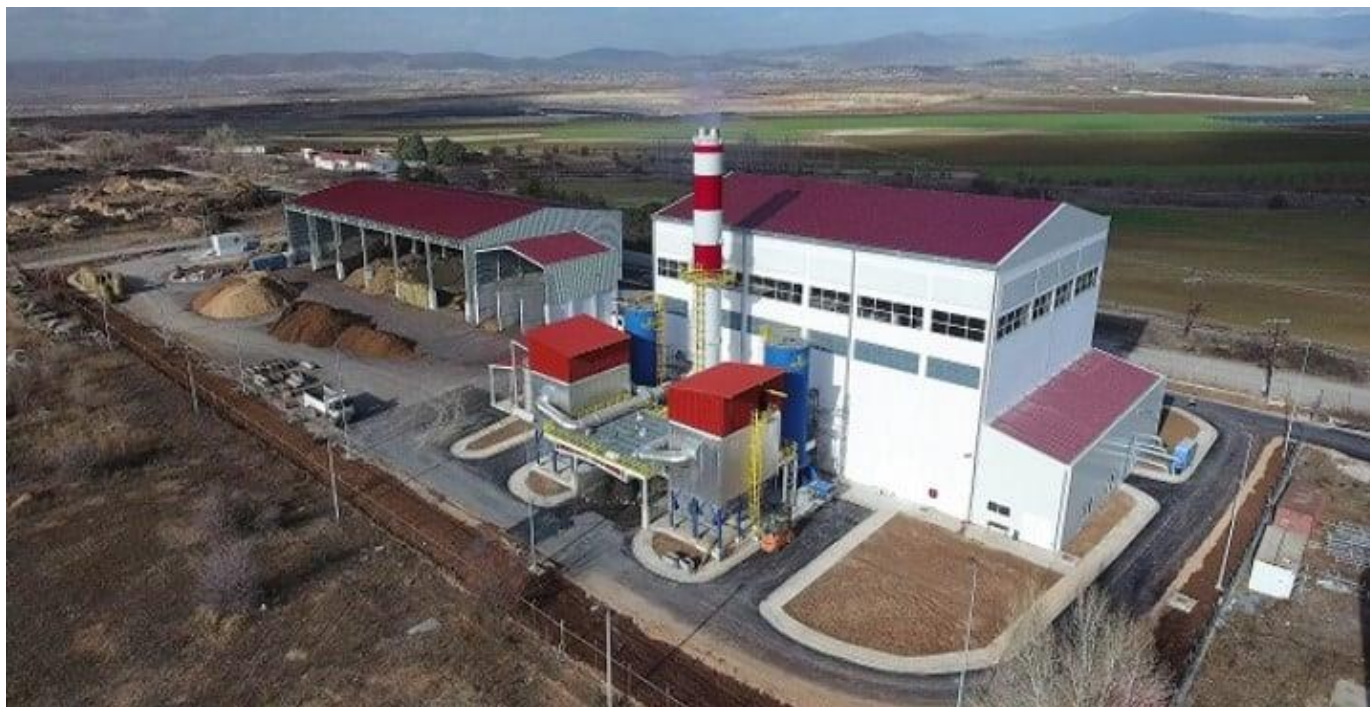
DETEPA 30 MWth district heating plant at Amyntaio Fuel: Biomass (wood chips, agropellets, maize residues), lignite
