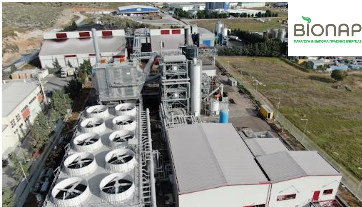
Viopar 5 MWe biomass plant at Volos Fuel: Exhausted olive cake, sunflower husk pellets, wood chips
